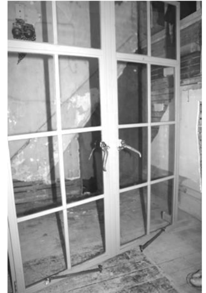
Window after restoration
