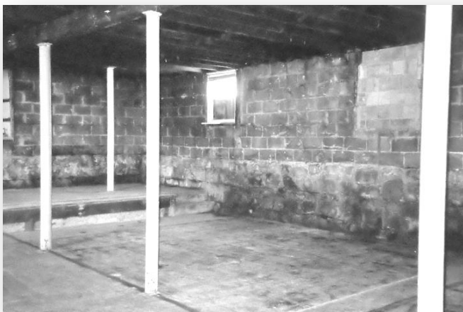
Lower Level before renovation
