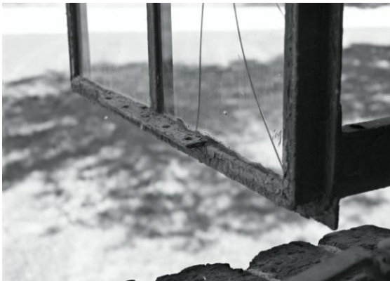
Window before restoration
